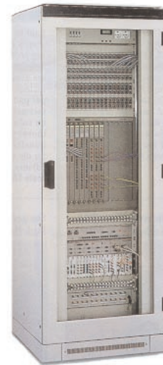
Figure 9: Typical telecom cabinet housing electronics equipment.
